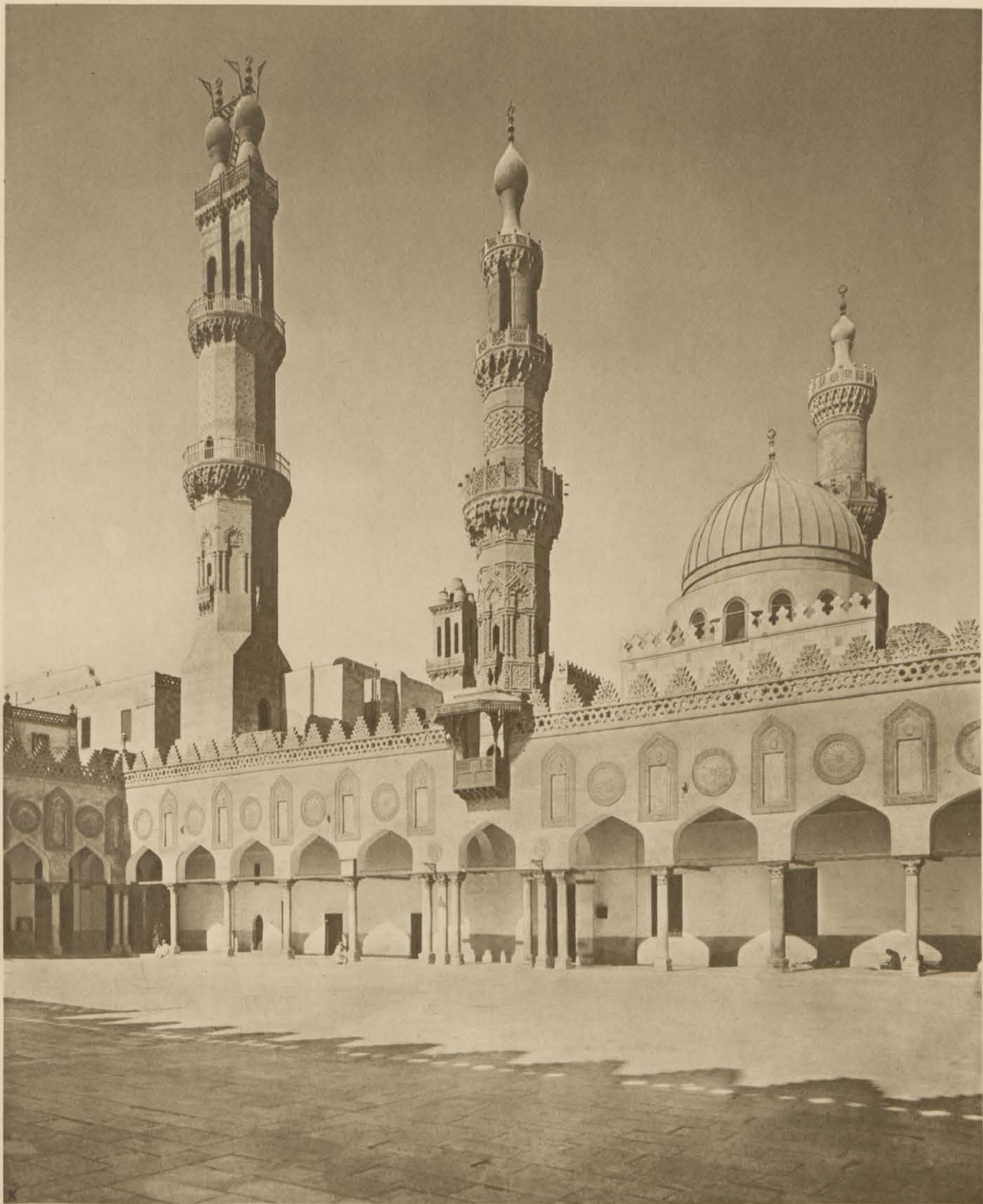
Courtyard, showing Minarets of Qāyt-Bāy and al-Ghūrī
