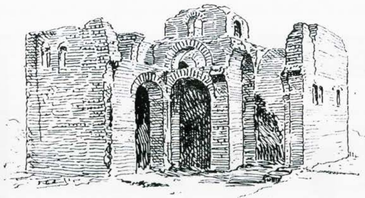
FIG. 13. Serre. South church from SW.
