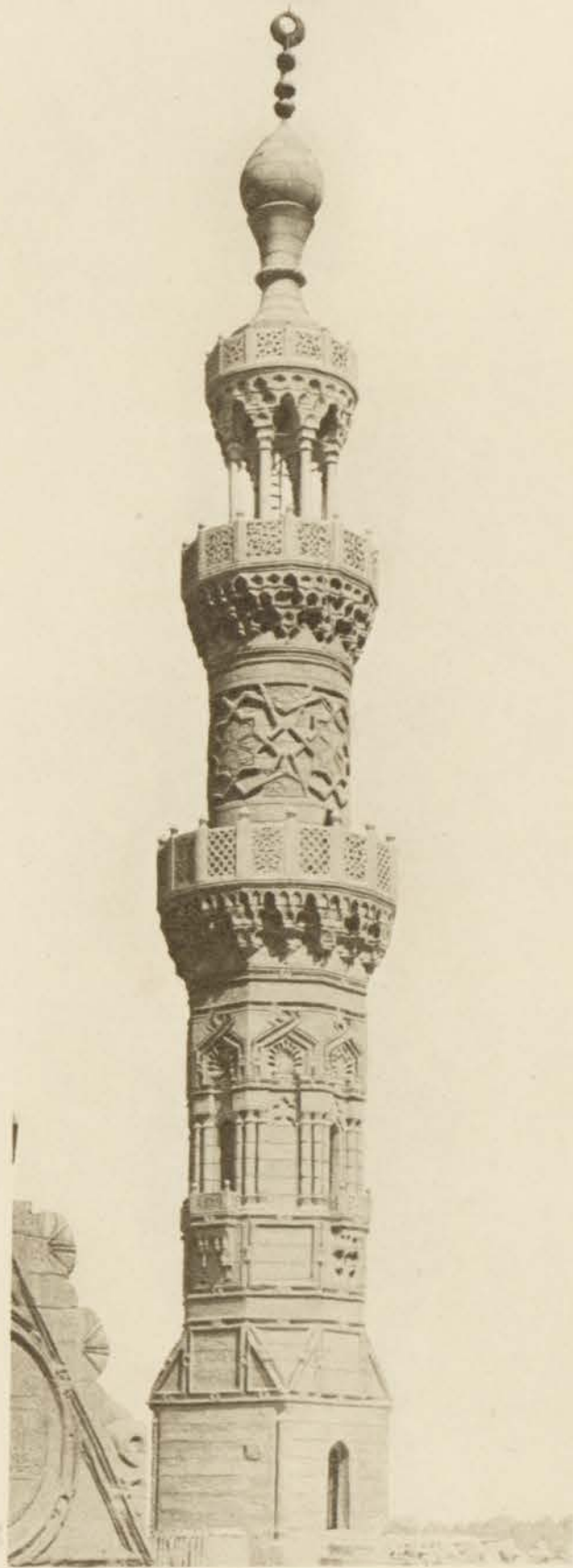
THE MOSQUE & KHĀNQĀH OF SULTAN QĀYT-BĀY (MAMLŪK CEMETERY)
