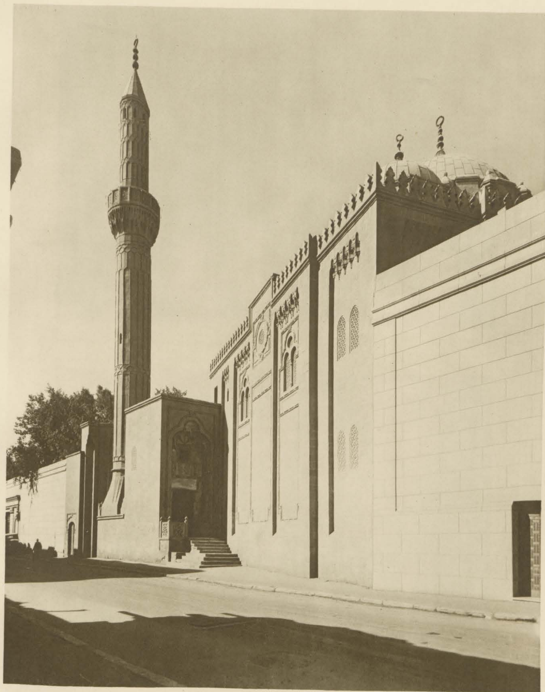
Exterior from the street
